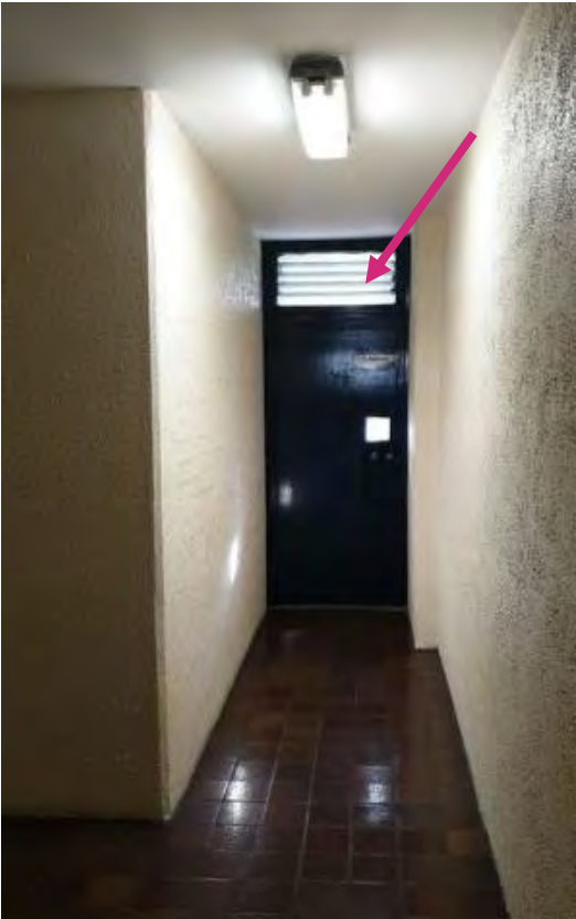
Figure 17: Stair/lift lobby vent (red arrow) for Staircase 24
